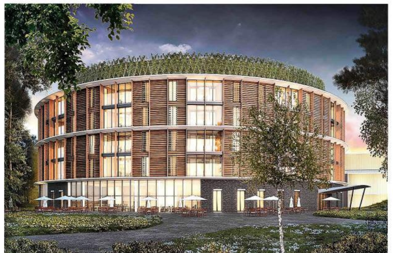
Das Bettenhaus soll 2019 fertig sein. • The ward building is to be completed in 2019.
